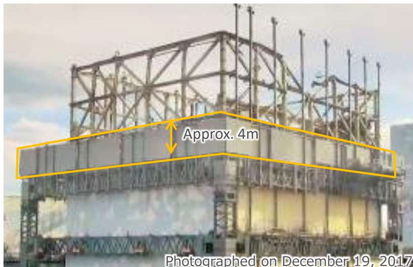
Wind prevention fence construction
