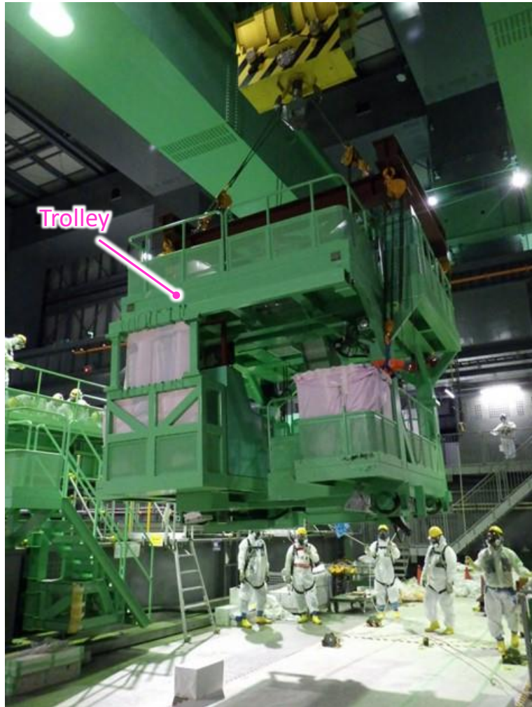
Hoisting the trolley (photographed on November 12, 2025)
