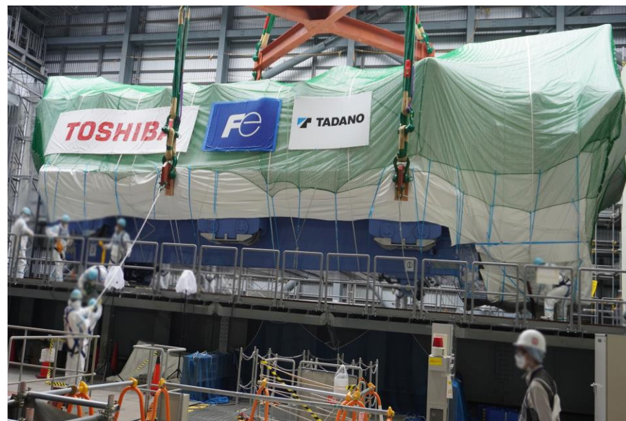
Affixing the fuel handling equipment to the girder rails at the fuel removal work platform (Photographed on May 30: some parts of the photo have been altered)
