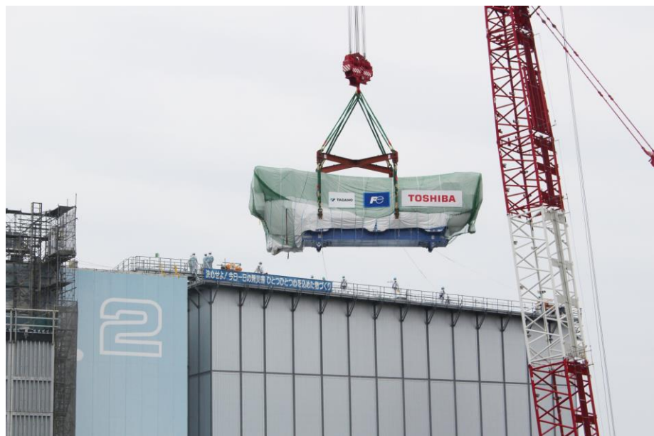
The fuel handling equipment hoisted by a crane (Photographed on May 30: some parts of the photo have been altered)
