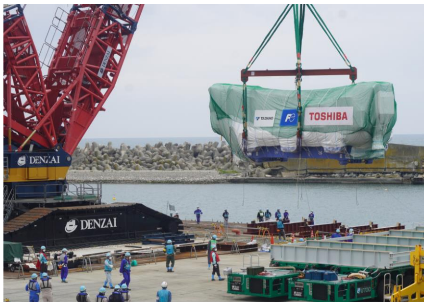
Unloading of fuel handling equipment (photographed on May 24: some parts of the photo have been altered)
