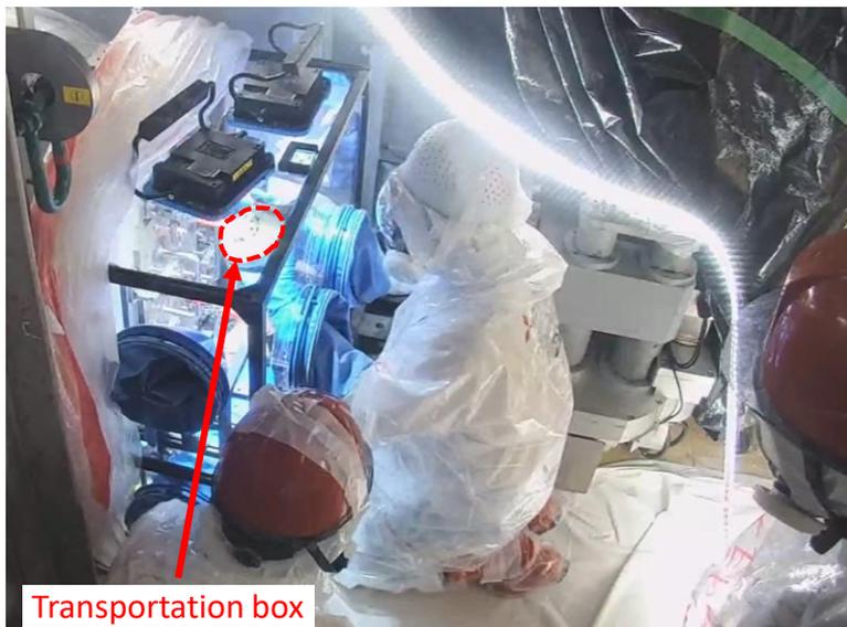
Removing the transportation box from the side hatch of the enclosure
