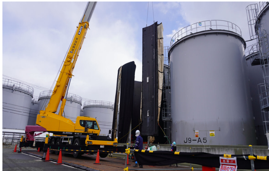
<Side plates from a tank in the J9 area being hoisted > (Photographed at around 2:10 PM on February 20)
