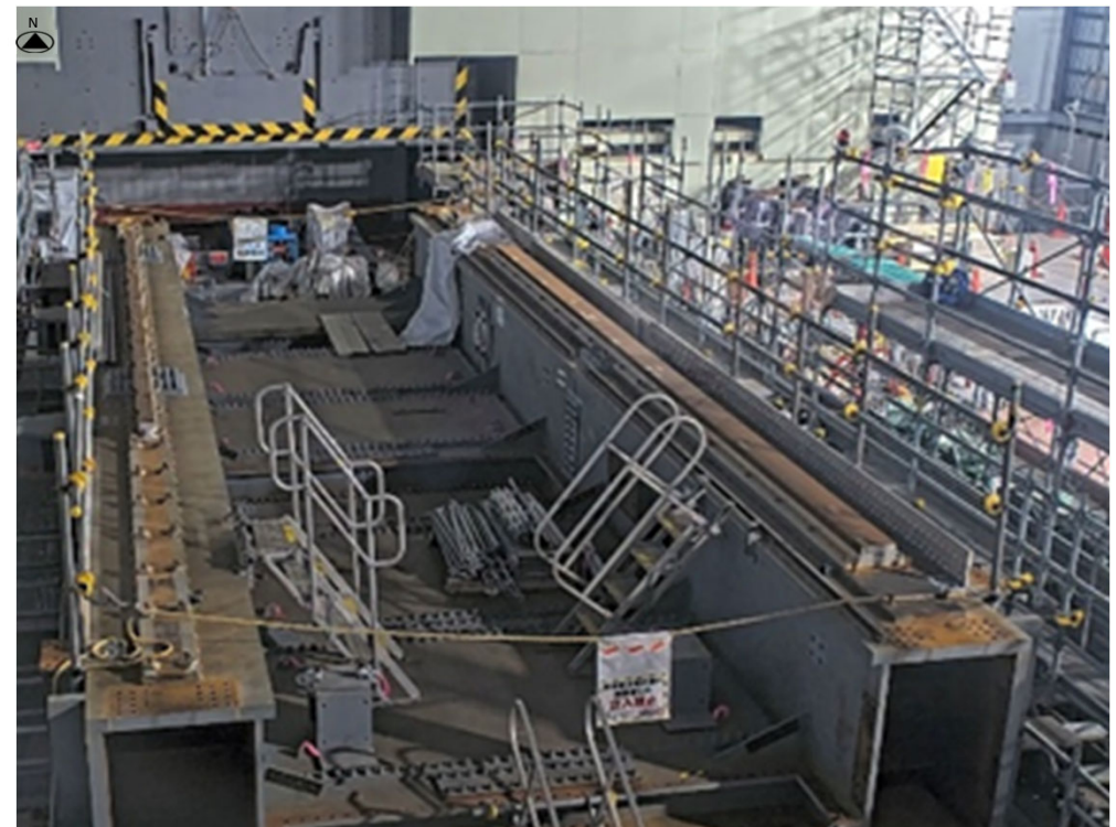
Runway girder framework installation (Photographed on December 13, 2024)
