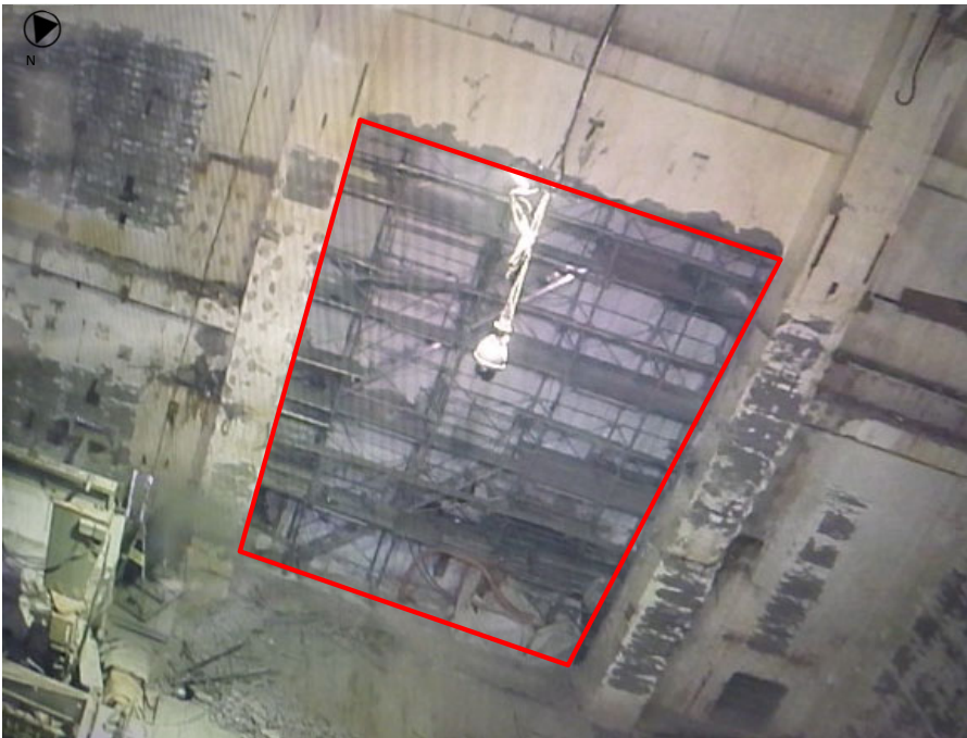
Photo①: Opening for the runway girder (Photographed on December 6, 2024)
