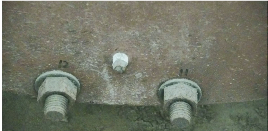
5. N 2 injection insertion line for flange leak tests
