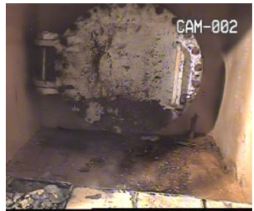
In front of the X-6 penetration ( After concrete block removal )
