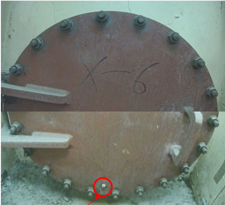
N 2 injection insertion line for flange leak tests
