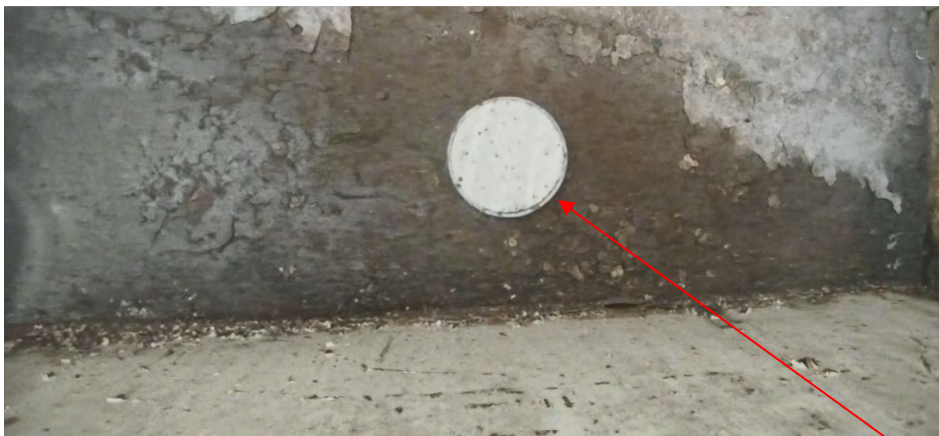
3. Floor (shield wall side)
