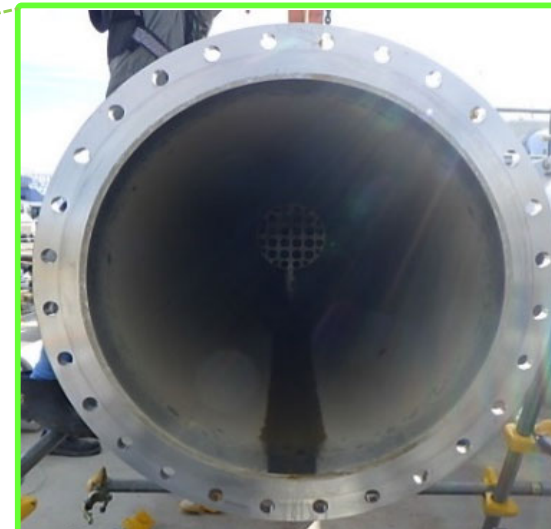
Main pipe (no corrosion)
