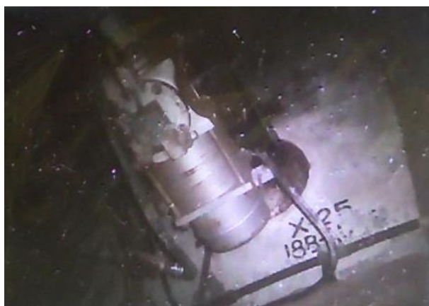
Photo 5 : Location C (Approximately 3m from the floor around the X-25 penetration)
