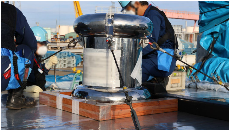
Off-site transport container loaded onto the off-site transport vehicle
