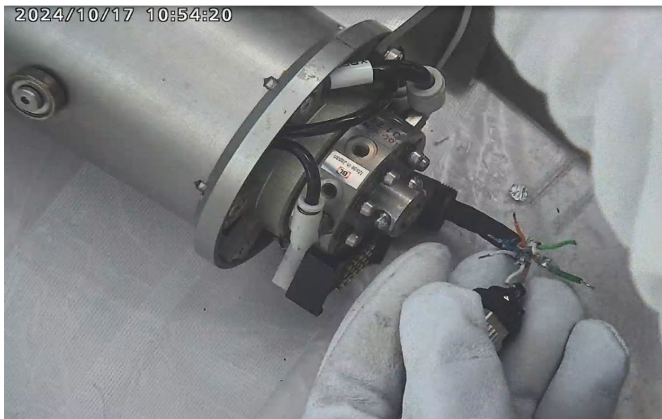
Working on the end jig monitoring camera (camera ①) (Photographed on October 17, 2024)
