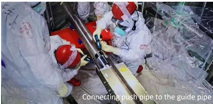
Trial retrieval work status (passing through the isolation valve)
