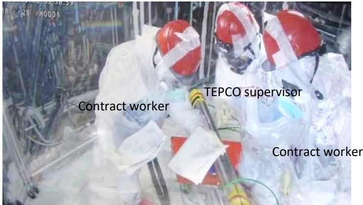
Rearranging push pipes in their correct order(field check)
