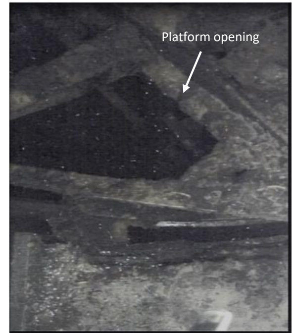
Footage from telescopic arm camera (Pedestal opening, platform opening conditions)
