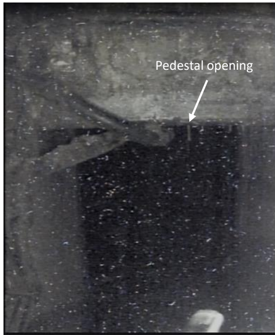
Footage from telescopic arm camera (Pedestal opening, platform opening conditions)
