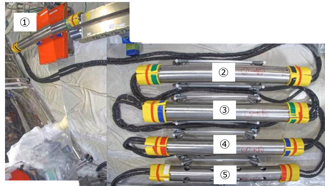
Completion of push pipes restoration work (September 8, 2024)
