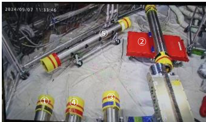
Rearranging push pipes in their correct order at the Fukushima Daiichi Nuclear Power Station site (Photographed between September 7-September 8, 2024)
