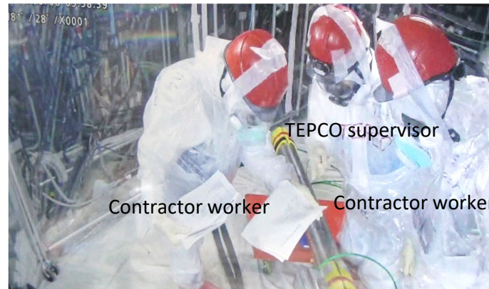
Rearranging push pipes in their correct order at the Fukushima Daiichi Nuclear Power Station site (Photographed between September 7-September 8, 2024)
