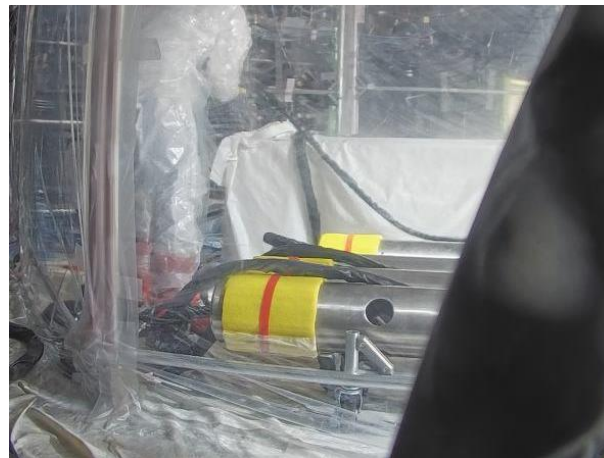
Inserting the cable into the push pipes
