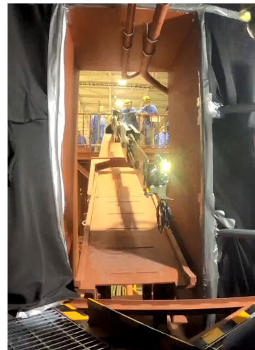
Inserting the equipment into the pedestal opening
