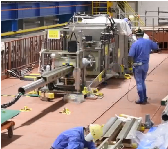
Inserting the guide pipe
