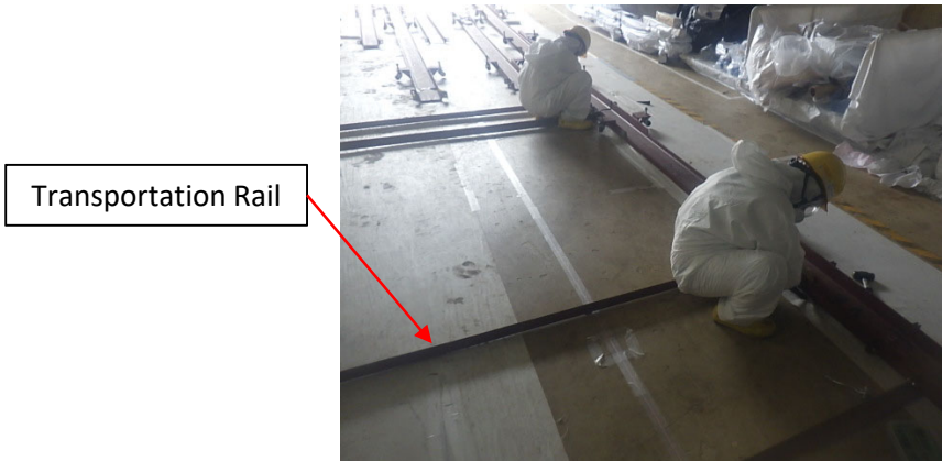
Installing transportation rail on July 18
