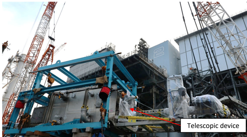
Carrying the telescopic device inside the reactor building on July 19
