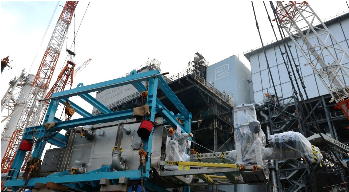
Carrying the telescopic device into the reactor building
