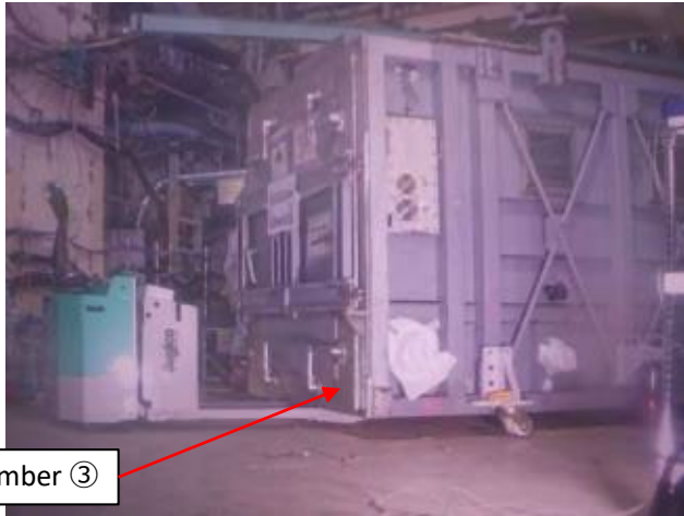
Removing the isolation chamber③
