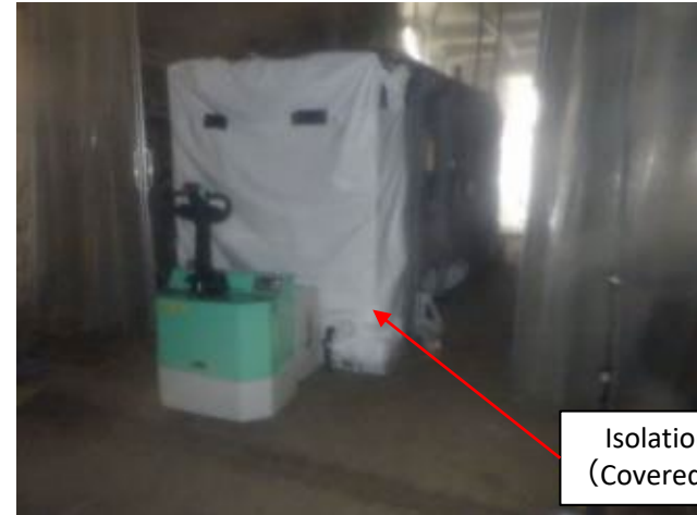
Carrying the isolation chamber ③ to the large freight entrance
