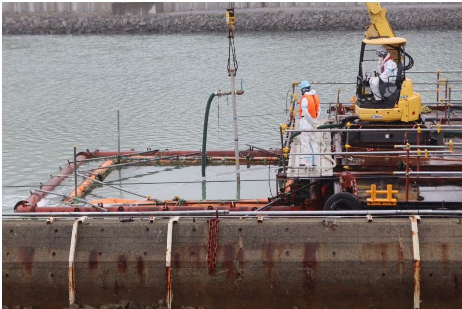
Figure 2. Seafloor re-covering construction (second layer of cover) (Photographed on May 16)
