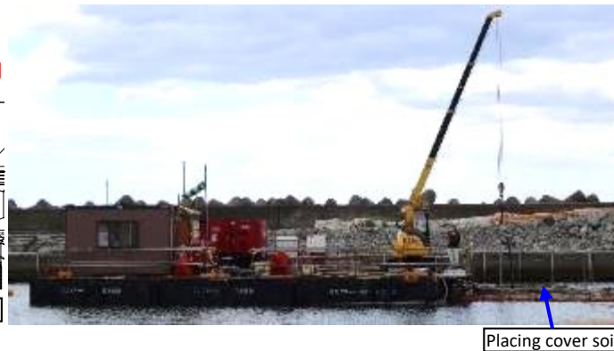
Figure 5. Laying soil for the second layer using the uni-float barge
