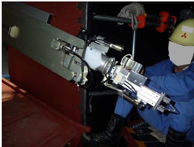
Inserting end jig into the pedestal
