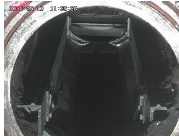
X-6 penetration after the removal of deposits
