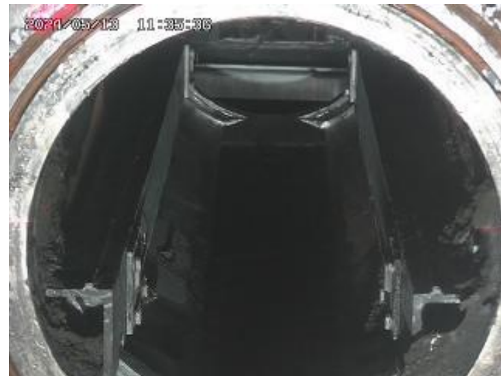
X-6 penetration (after the removal of deposits)
