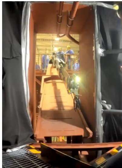
Inserting the equipment into the pedestal opening
