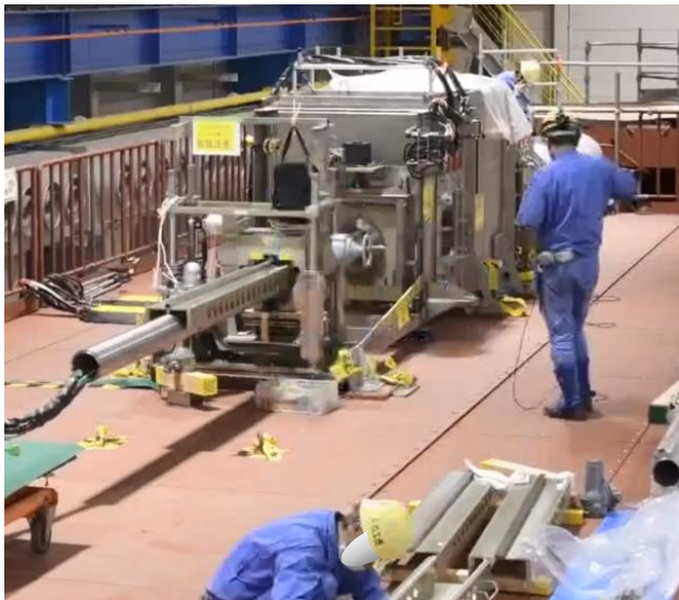
Inserting the guide pipe
