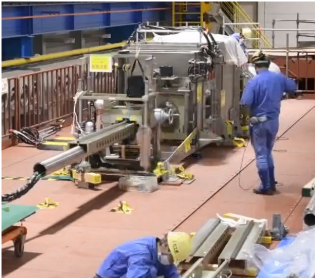
Inserting the guide pipe
