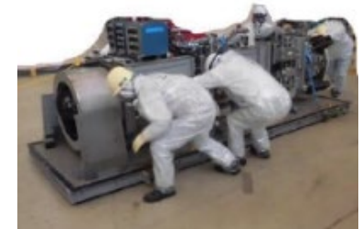
Removal of deposit removal equipment (low pressure water)
