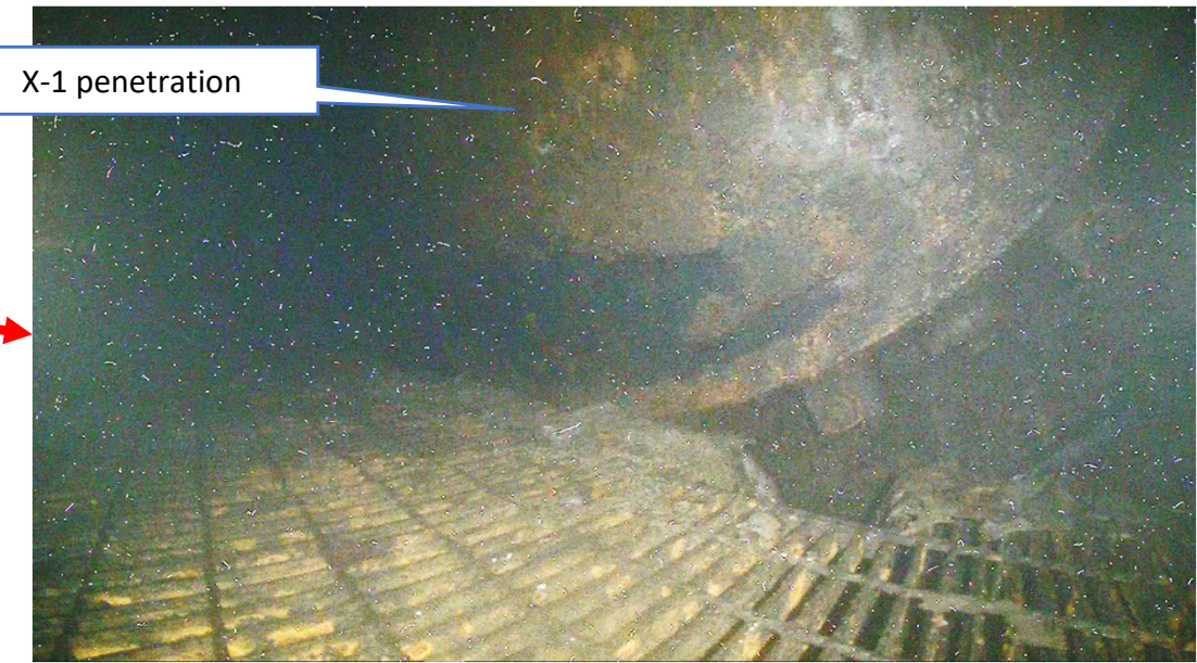
Photo 1. X-1 penetration condition
