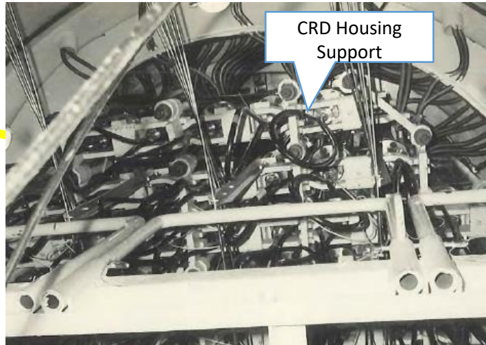
Photo 2. Looking up toward the upper pedestal (at the time of construction)
