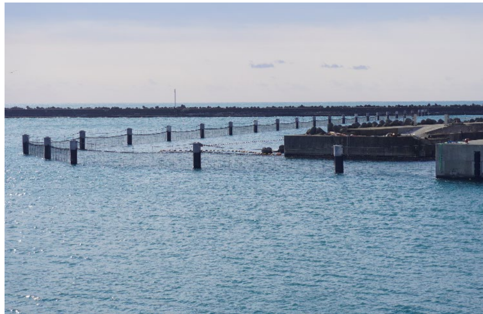
Figure 2-2. The net surrounds the outlet to the Units 1-4 intake open channel
