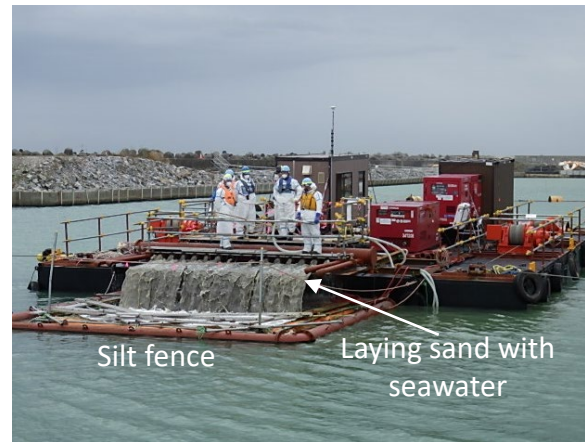
Figure 10. Laying sand for the first layer using the uni-float barge
