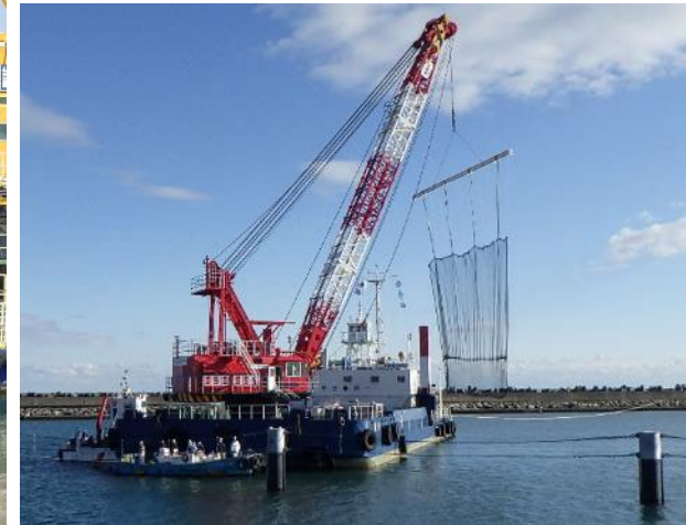
Figure 5. Crane ship used to install the high durability net (Photo taken on January 10, 2024)
