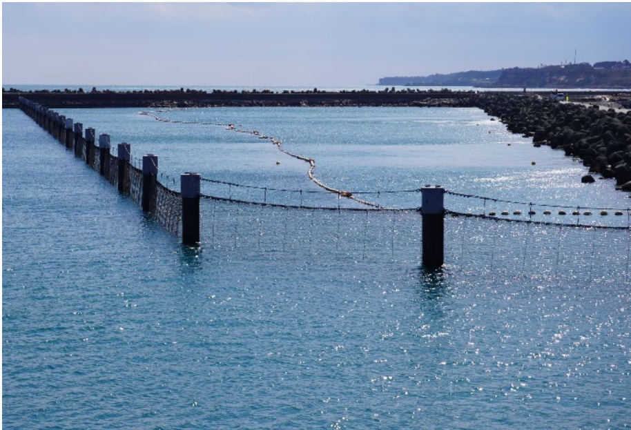
Figure 2-1. The net surrounds the east sea wall and the Units 1-4 intake open channel
