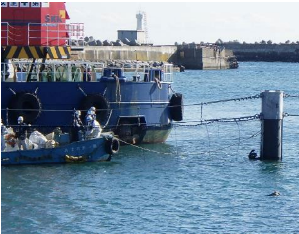
Figure 6. Workers installing the high durability net (Photo taken on January 10, 2024)
