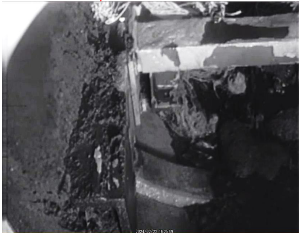
After spraying with high-pressure water (bottom left of the X-6 penetration)
