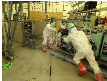
Installation of deposit removal equipment (low pressure water)
