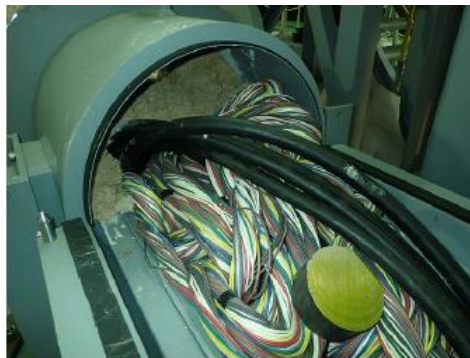
Conditions inside the X-6 penetration (mockup)
