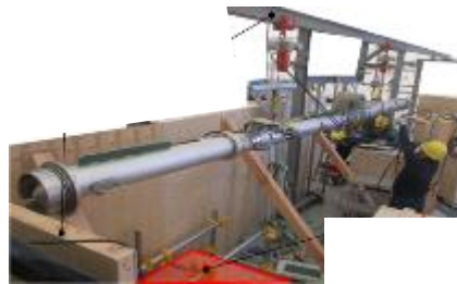
Spray jig installation ※Connected to X-53 penetration
