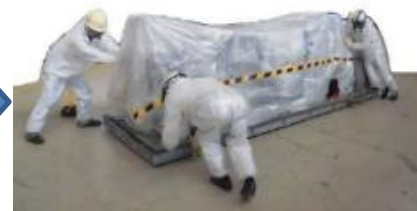
Removal of deposit removal equipment (high pressure water, abrasive water jet)
