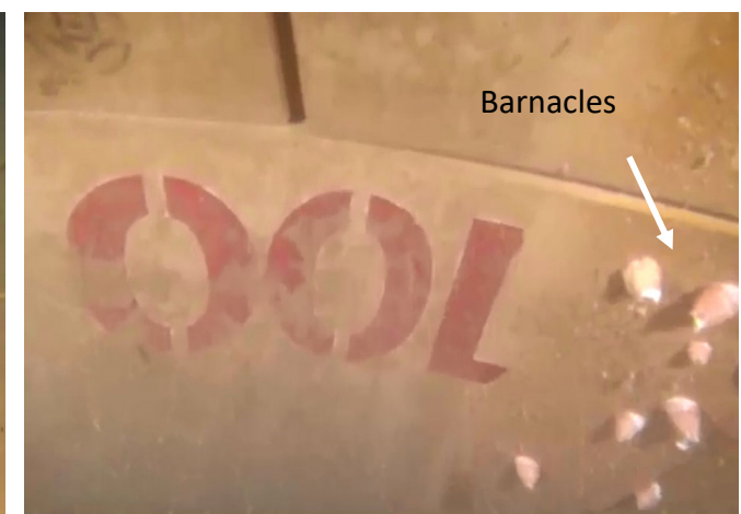
Top of tunnel approximately 100m from the downstream storage
