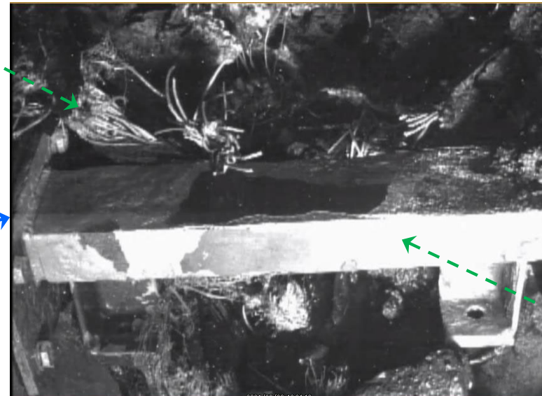
X-6 penetration (After the deposit removal work by high pressure water spray ①)
