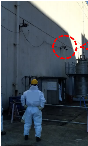
【Field conditions (external view of the building)】
