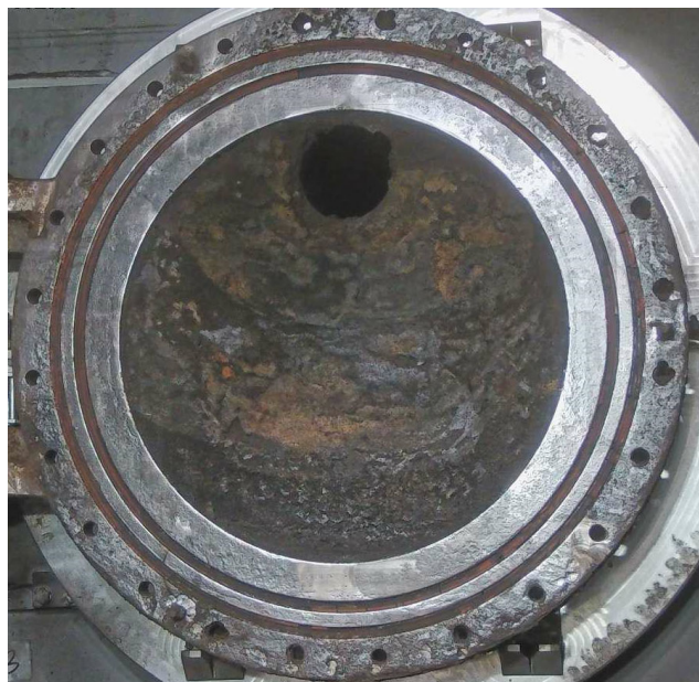
X-6 penetration (Before the deposit removal work)
