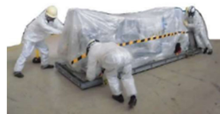
Removal of deposit removal equipment (high pressure water, abrasive water jet)
