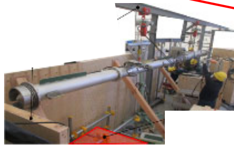
Spray jig installation ※Connected to X-53 penetration
