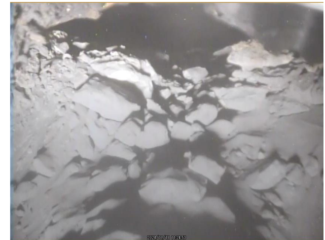
After the work on January 18
