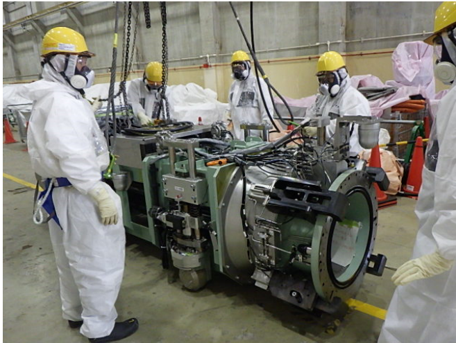
Exterior view of the deposit removal equipment (low pressure water)
