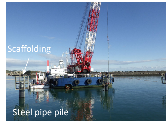
Attaching guiderails (hoisting)
