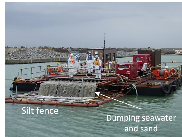
Dumping overlaying sand from the uni-float barge
