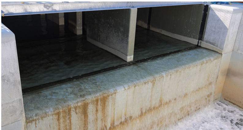
ALPS treated water diluted with seawater overflowing from the upper-stream storage to the down-stream storage
