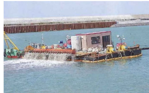
Figure 3. Using a uni-float barge for sand overlaying work
