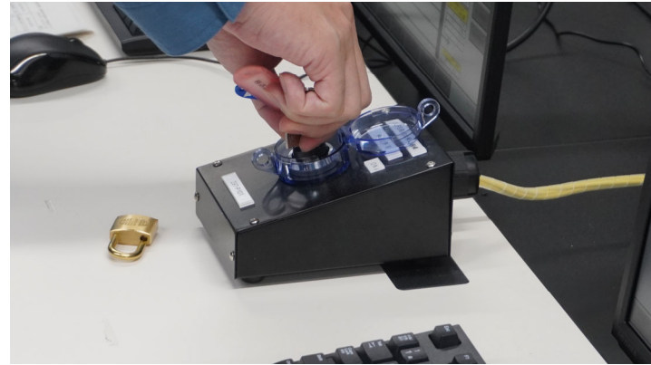
Key switch operations during the First Stage
