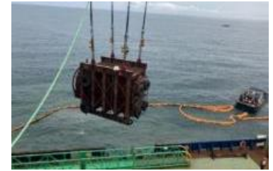
Removal of the shield machine
