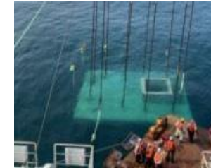
Installing the discharge outlet lid
