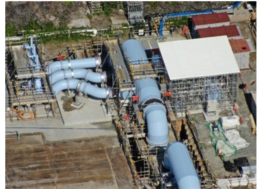
Installment of seawater transfer pipes and seawater pipe header
