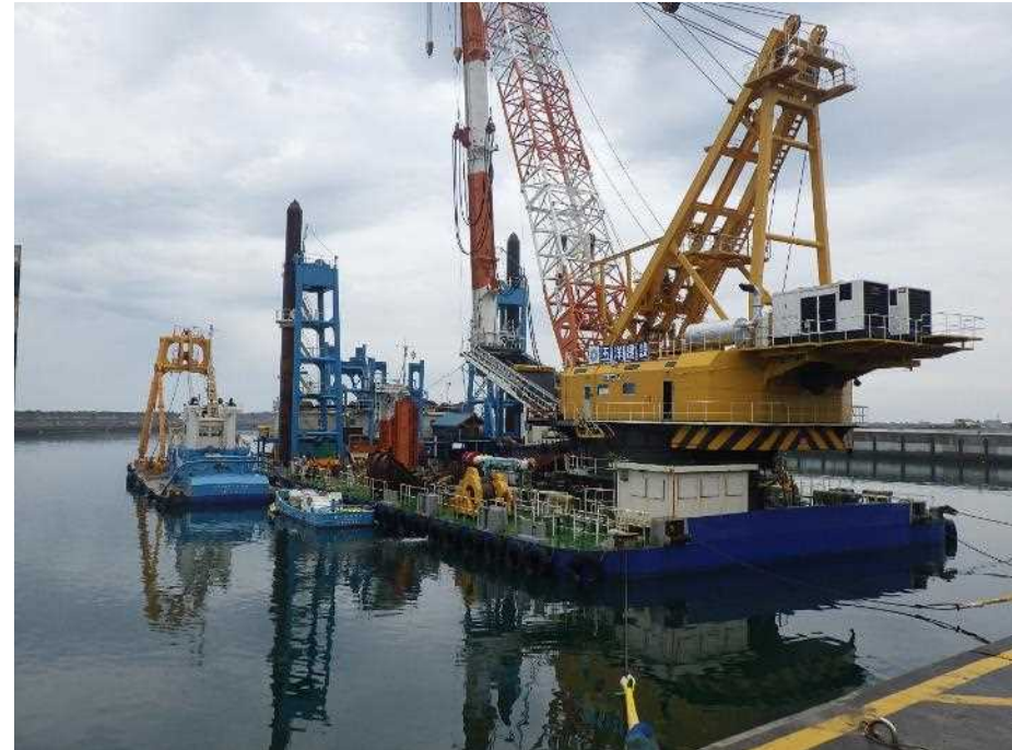
Figure 2. Construction ship (moored at the unloading wharf)
