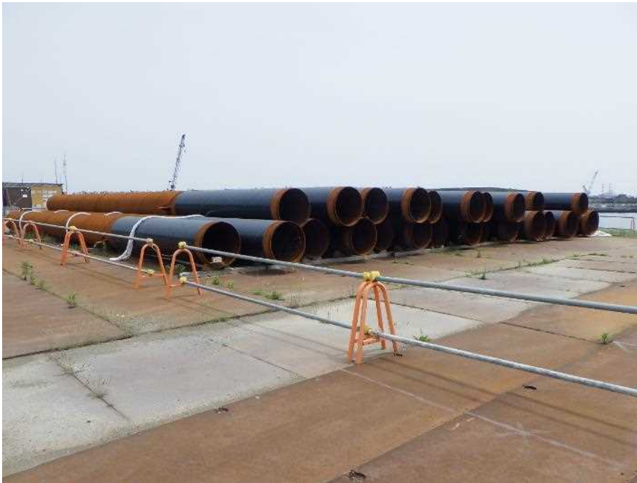
Figure 1. Steel pipe piles (Temporary placement on site)
