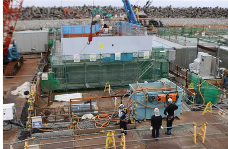
Discharge vertical shaft (down-stream storage)
