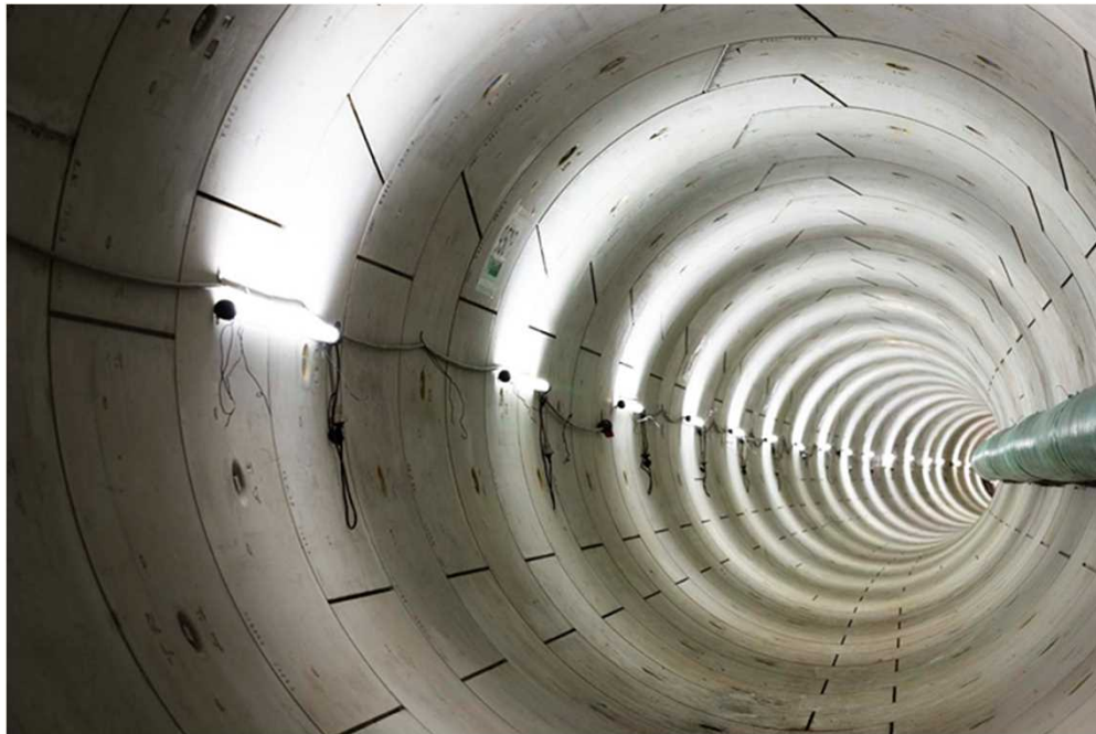
Inside the tunnel
