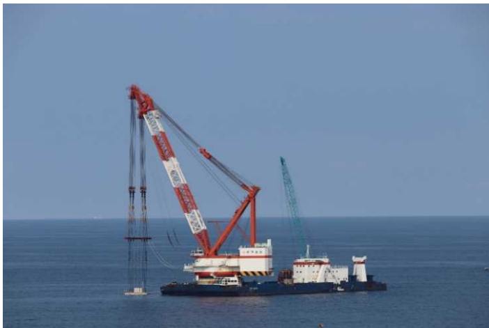
Discharge lid installation ①
