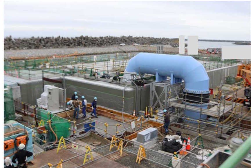
Discharge vertical shaft (upper-stream storage)
