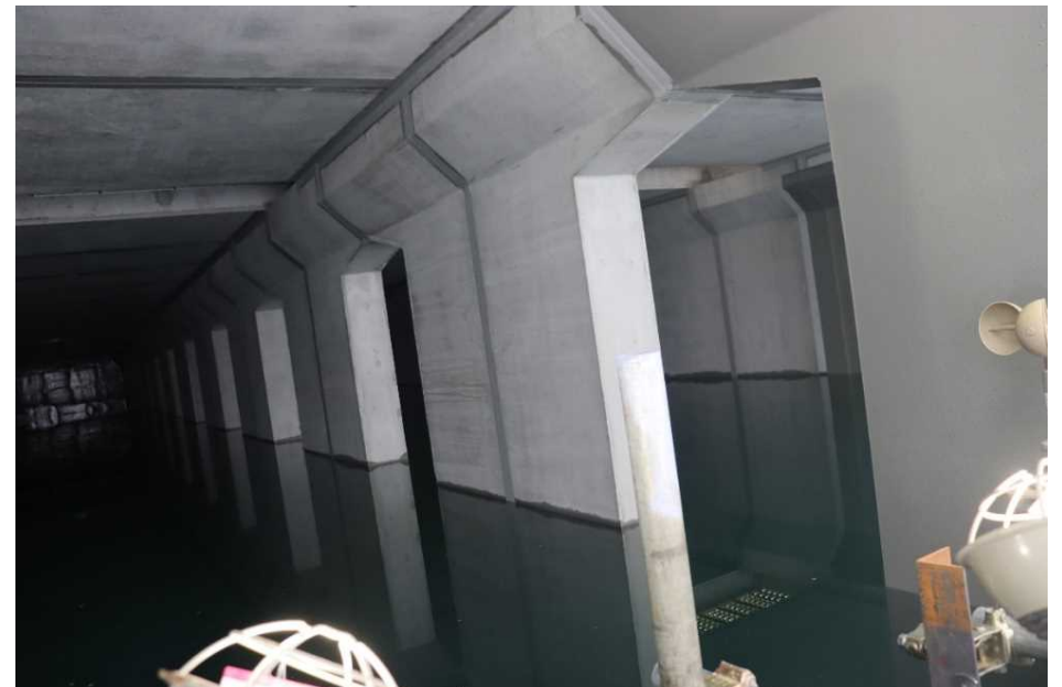
Picture of inside (After filling water)
