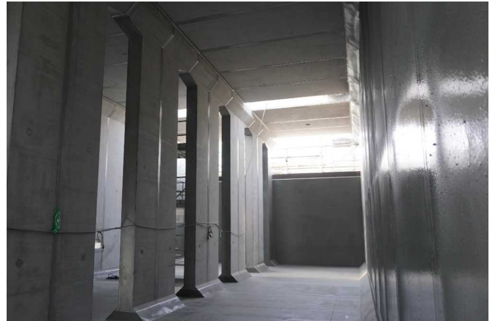
Picture of the inside (After applying waterproof sealant)
