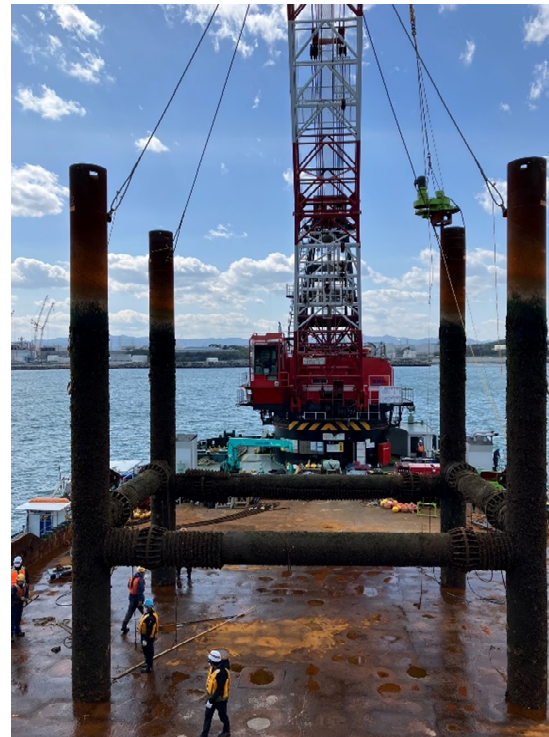
Guiding scaffolds (upper half) being removed
