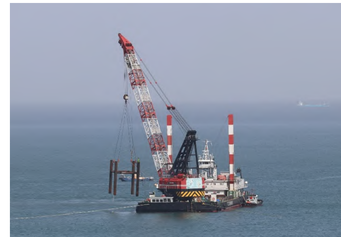
Guiding scaffolds (lower half) being removed
