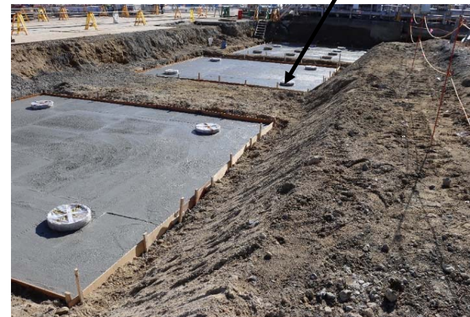
Building the seawater transfer pipe foundation
