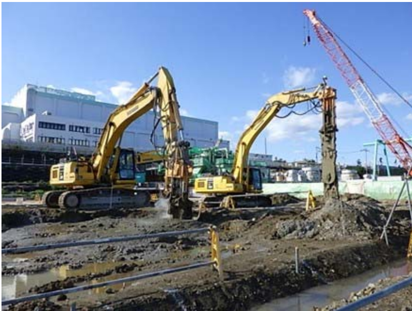
Ground improvement work
