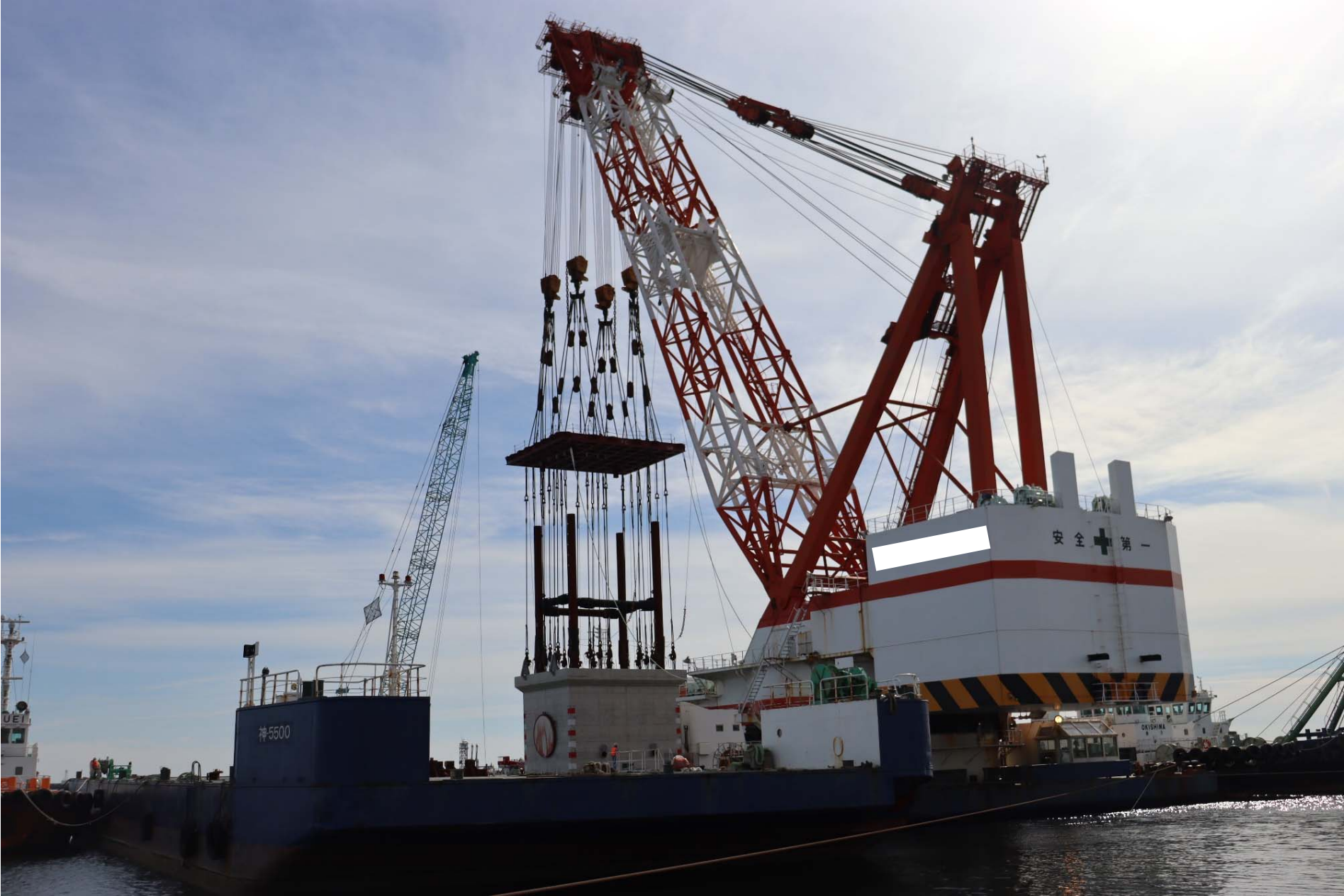
Caisson loading (November 17, 2022)
