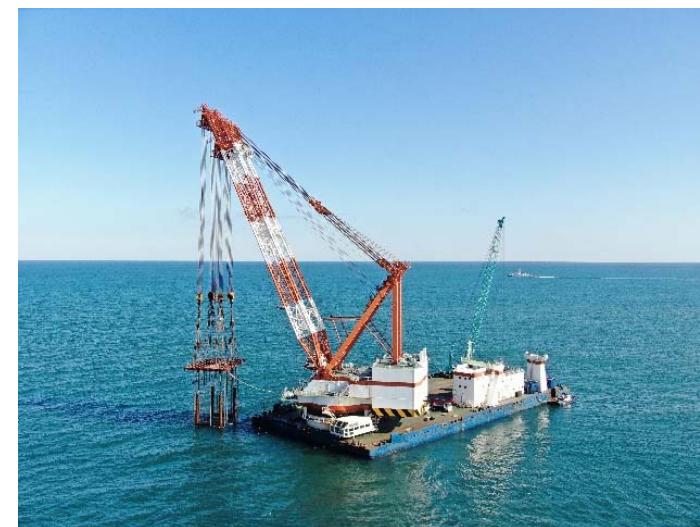
Construction of installing discharge outlet caisson ④
