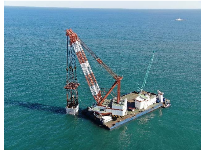
Construction of installing discharge outlet caisson ③
