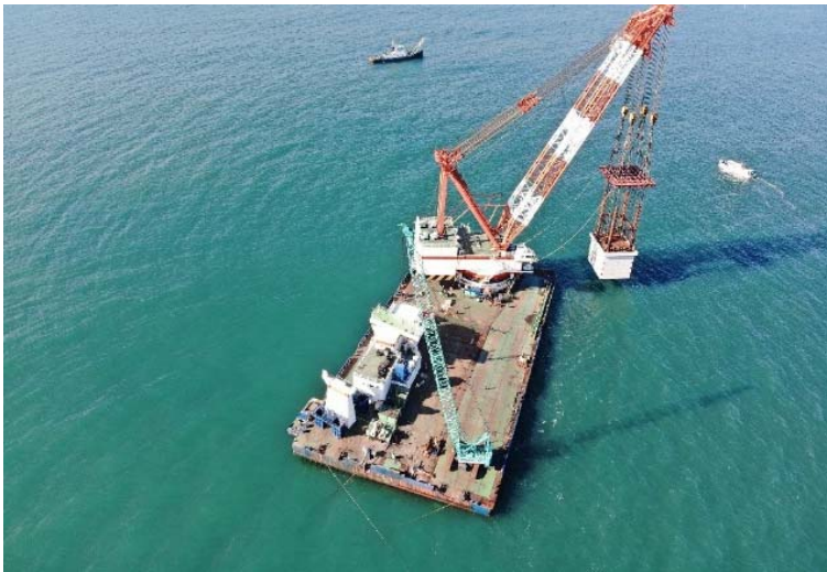
Construction of installing discharge outlet caisson ①
