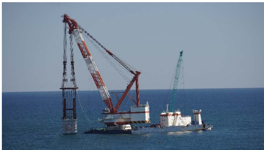
Construction of installing discharge outlet caisson ②
