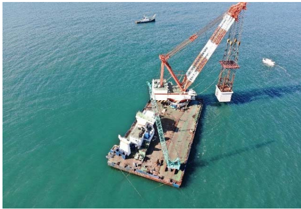
Construction of installing discharge outlet caisson ①
