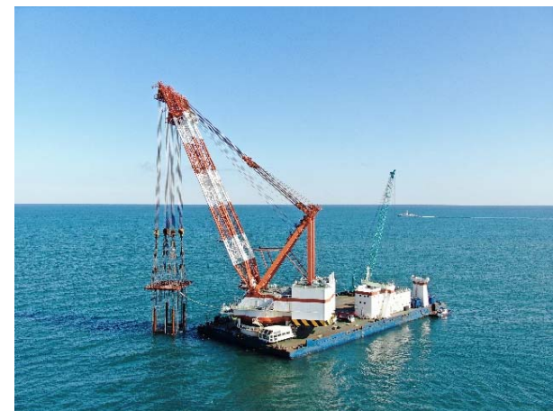
Construction of installing discharge outlet caisson ④
