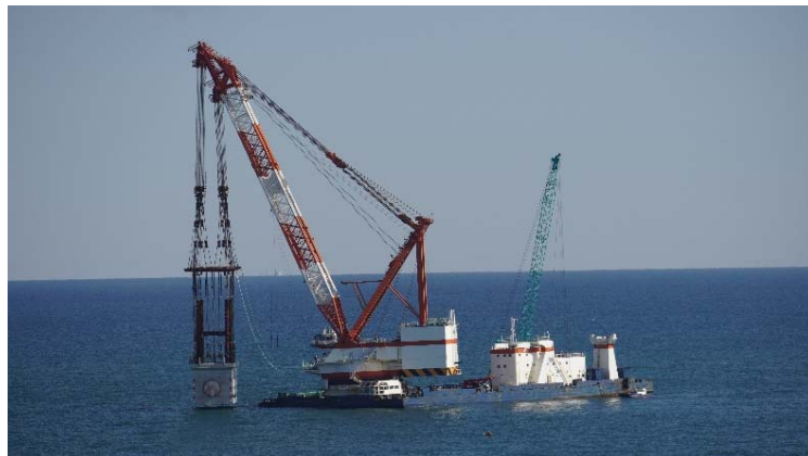
Construction of installing discharge outlet caisson ②
