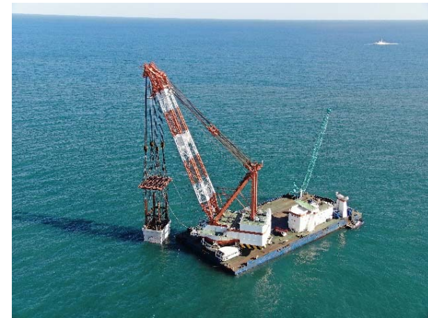
Construction of installing discharge outlet caisson ③
