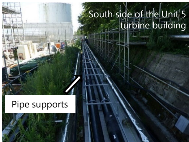
Transfer pipe support installation
