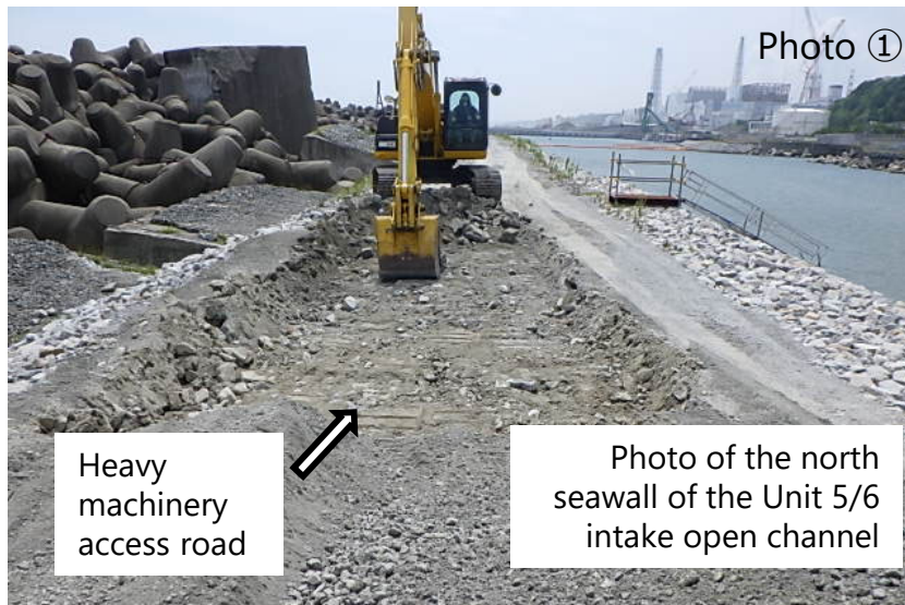
Heavy machinery access road construction
