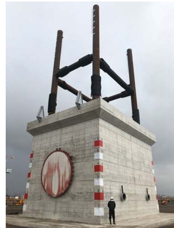
Discharge outlet caisson
