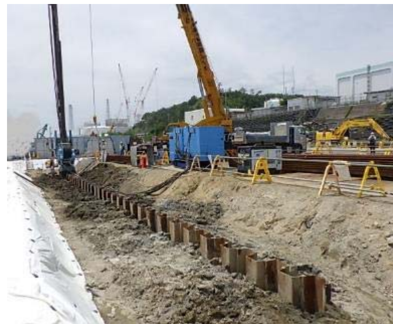
Retention wall construction
