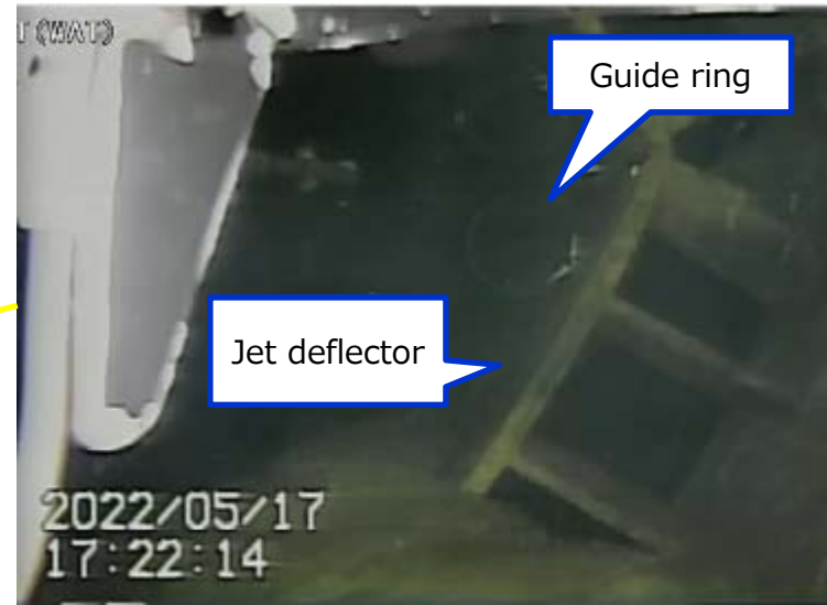
Photo 1. Looking down on jet deflector (E)
