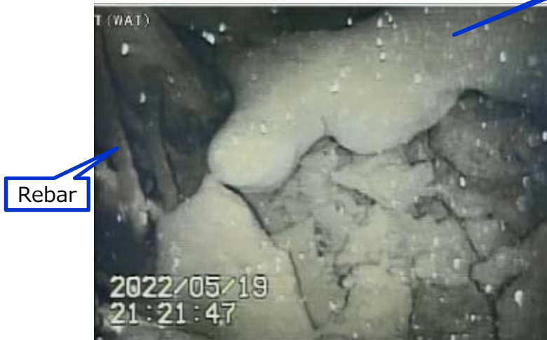
Photo 2. Conditions at the pedestal opening (inside nearest to the ROV)
