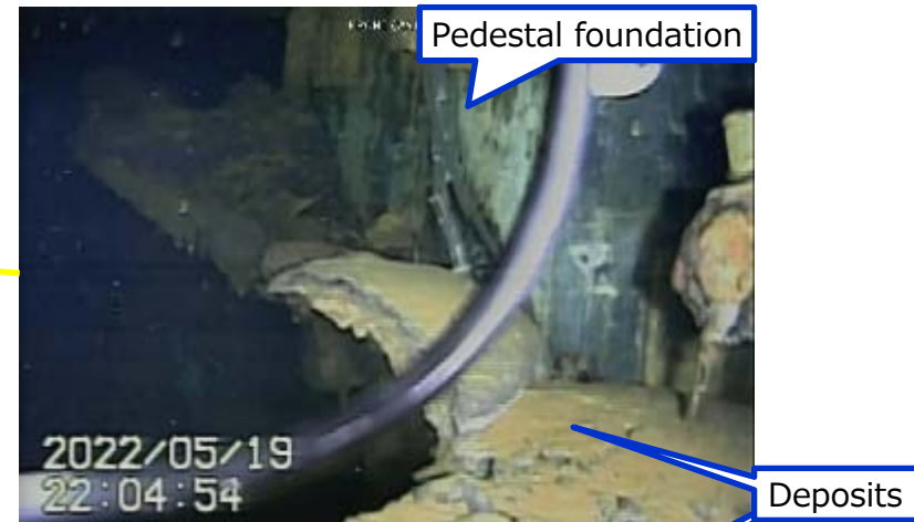
Photo 1. Conditions above the deposits at the opening of the pedestal (right side foundation)
