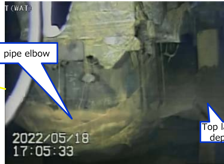
Photo 1. PLR (A) pipe conditions
