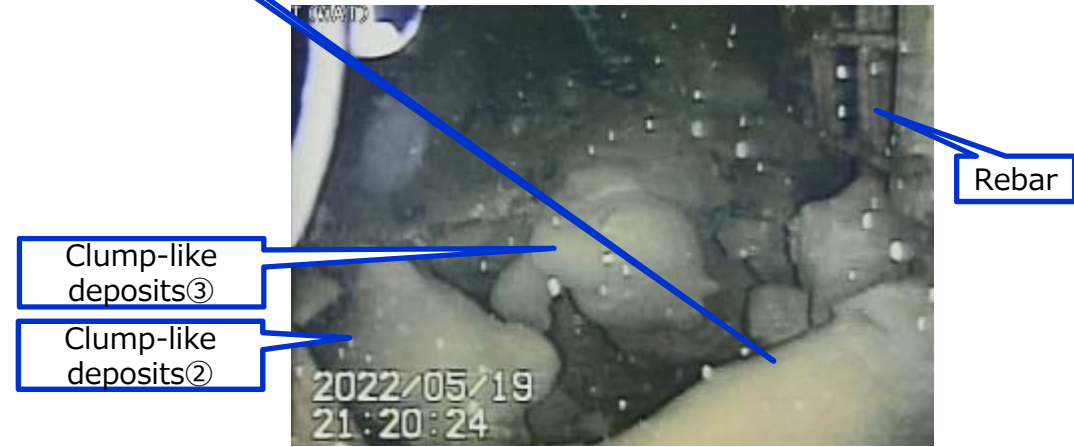
Photo 3. Conditions at the pedestal opening (inside nearest to the ROV)
