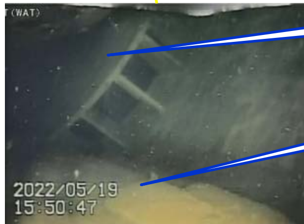
Photo 2. Looking down on jet deflector (C)
