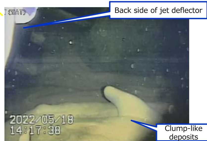
Photo 3. Conditions at the back of jet deflector (E)
