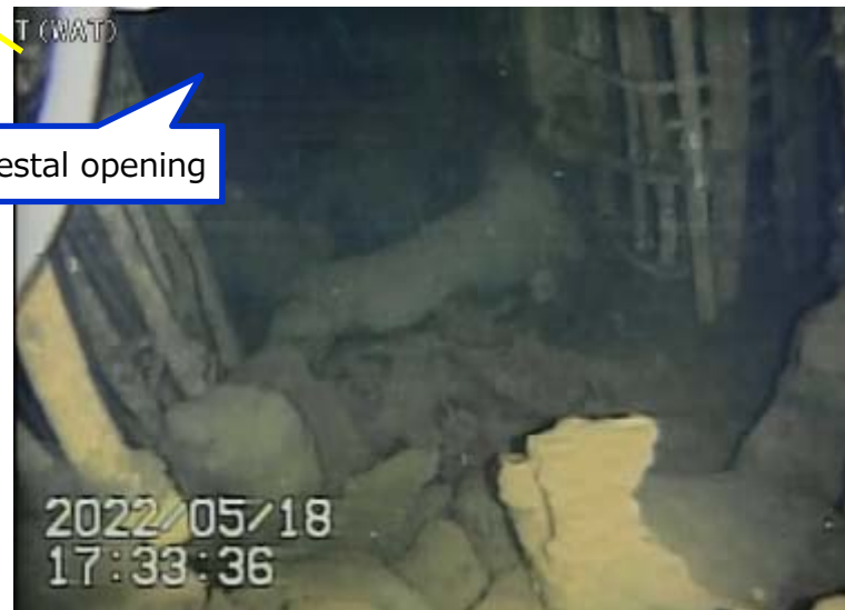
Photo 3. Deposits in front of the pedestal opening
