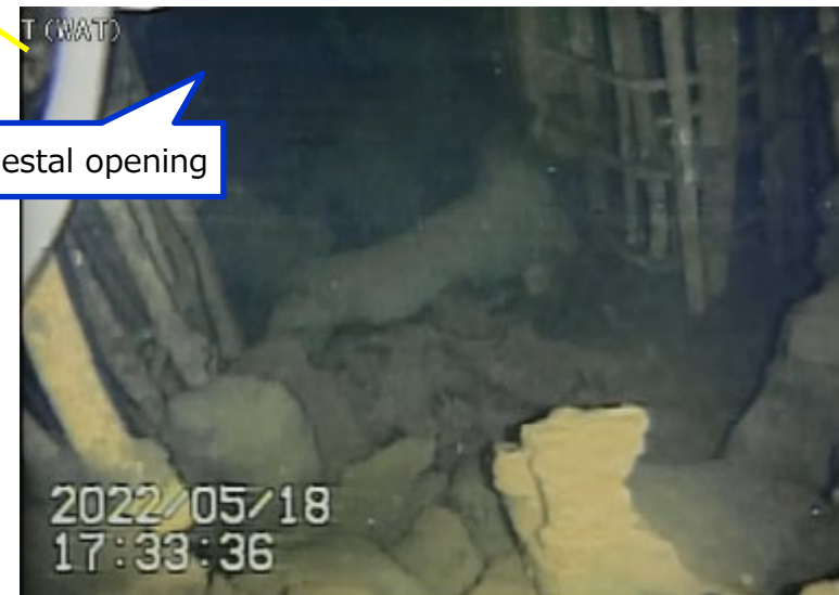
Photo 3. Deposits in front of the pedestal opening
