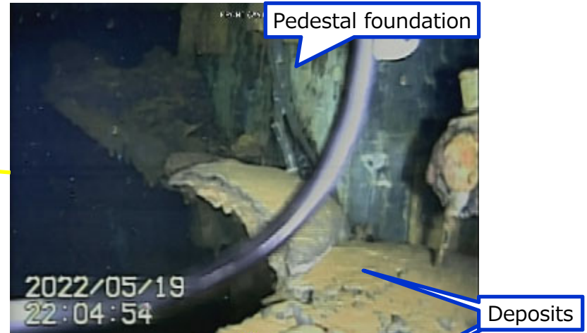
Photo 1. Conditions above the deposits at the opening of the pedestal (right side foundation)
