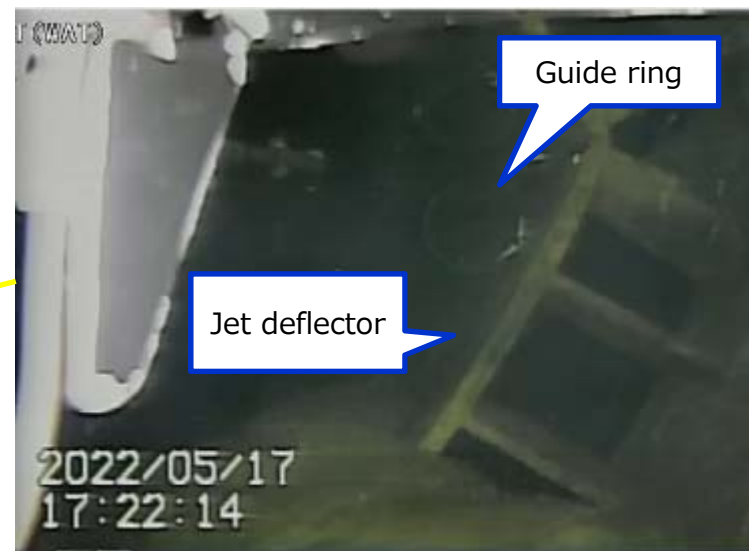
Photo 1. Looking down on jet deflector (E)
