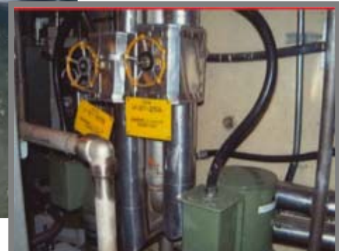
RCW pipe/valve Top layer of deposits (Reference photo) conditions prior to the accident in 2011
