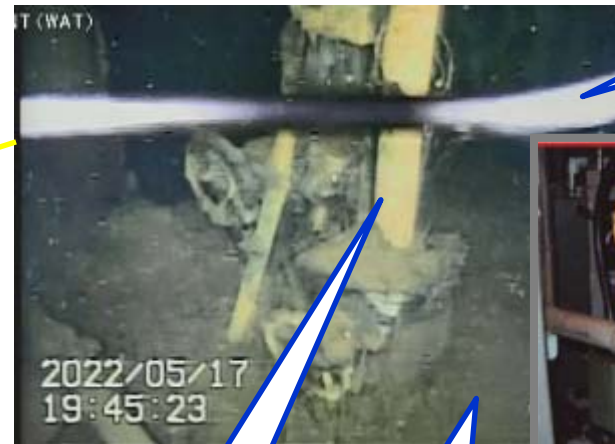
RCW pipe/valve Top layer of deposits (Reference photo) conditions prior to the accident in 2011
