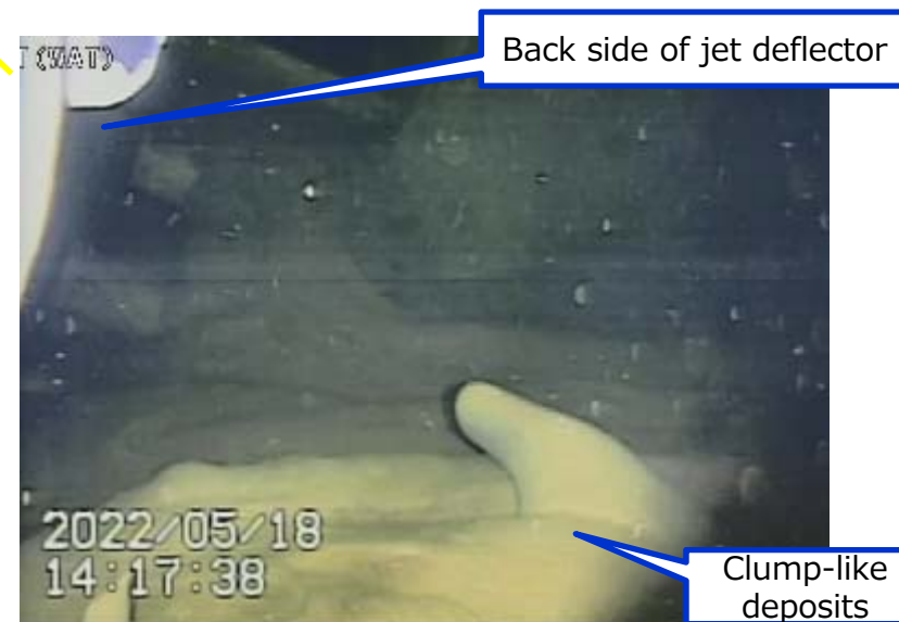
Photo 3. Conditions at the back of jet deflector (E)
