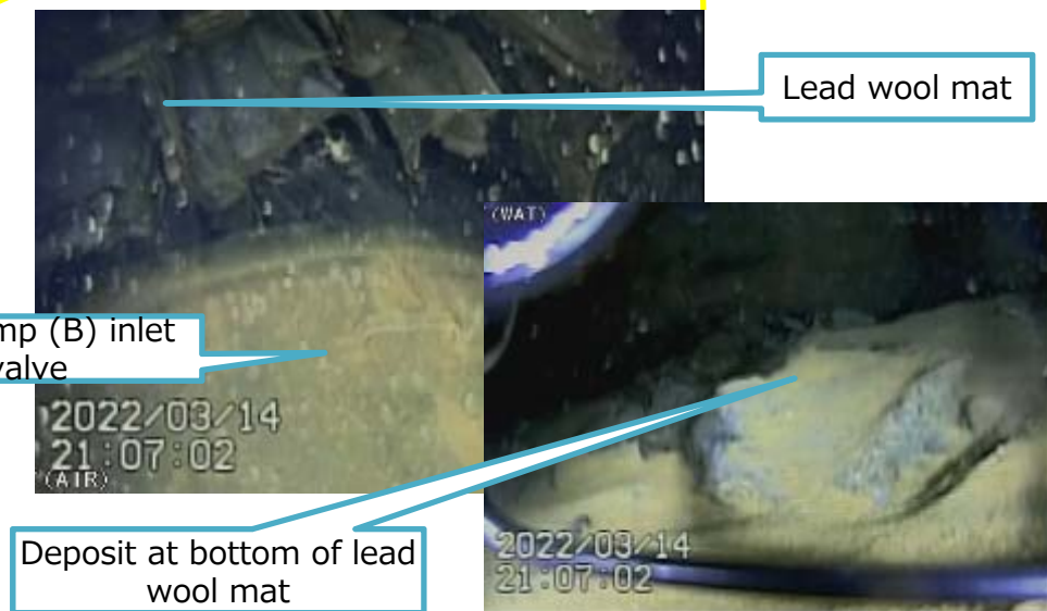
Photo 3. Conditions near PLR pump (B) inlet valve
