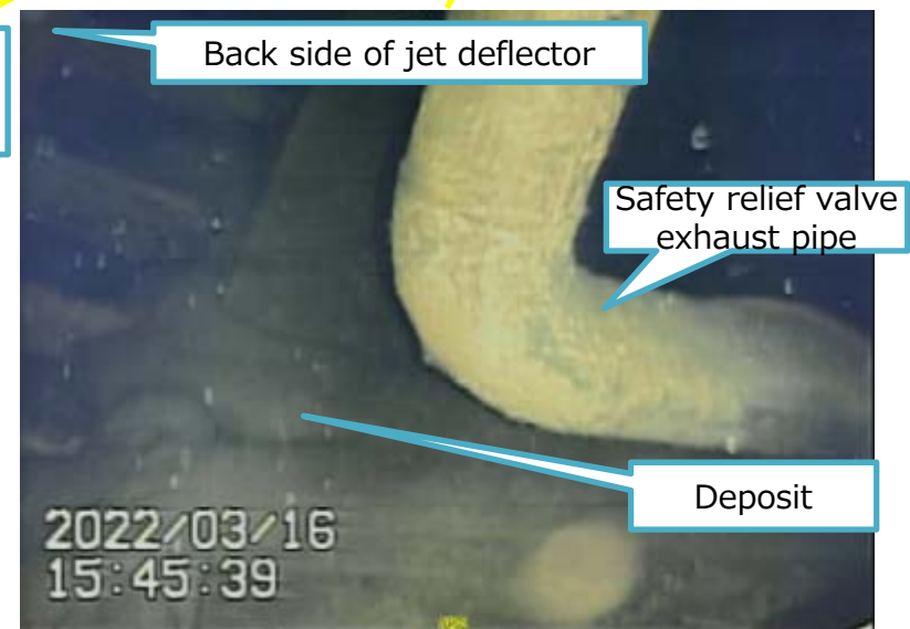
Photo 3. Conditions behind jet deflector (F) ② 9
