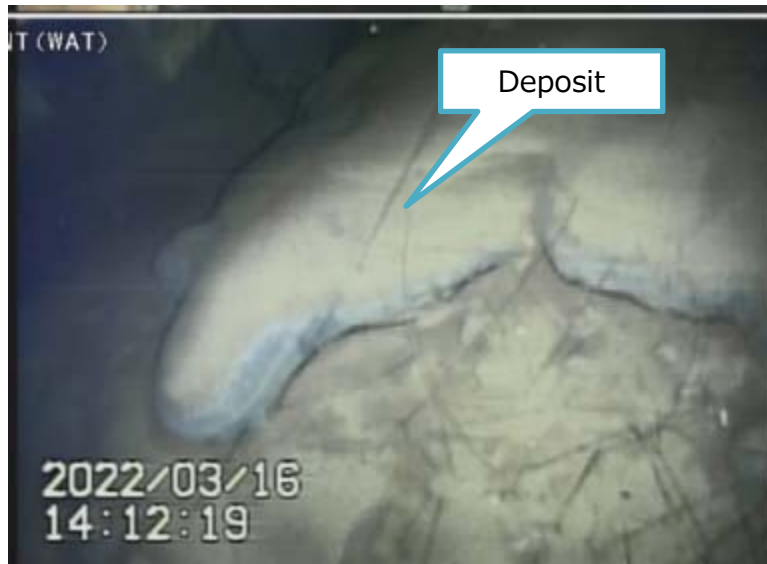
Photo 2. Conditions near jet deflector (F)
