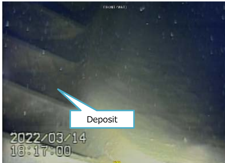
Photo 2. Conditions behind jet deflector (H) ②
