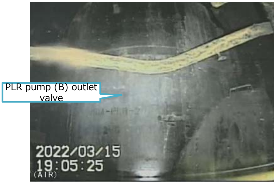
Photo 1. Conditions near PLR pump (B) outlet valve
