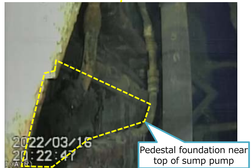
Photo 3. Conditions near pedestal foundation② 10
